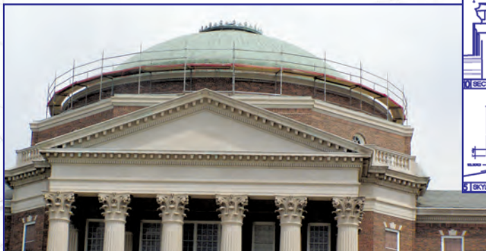
Completed project prior to the scaffolding's coming down.
