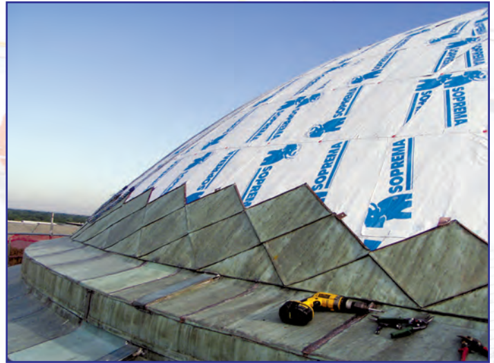
Waterproofing dome with diamond tiles being reinstalled.
