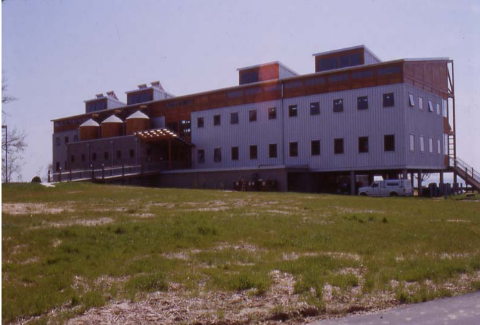
Photo 1. Entry side of the Philip Merrill Center Building shows the rain water capture system in the round towers.
