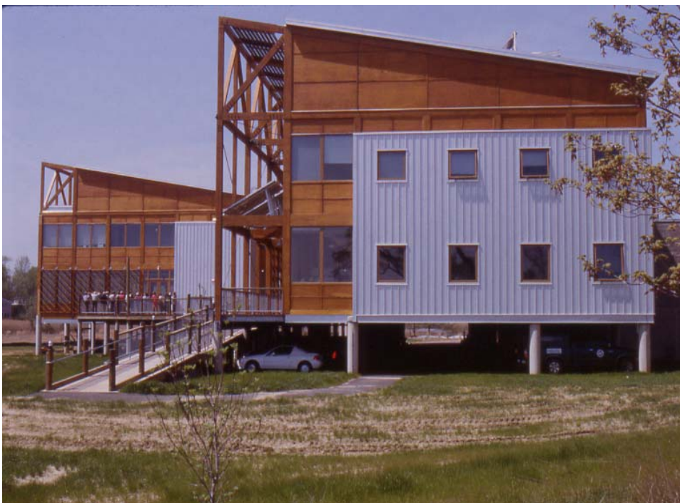
Photo 2. East side of the building with the Conference Center and outdoor deck on the far left. Shading devices on the south side of the building enclose an external walkway. Photo voltaic arrays can be seen on the sloped part of the shading device.
