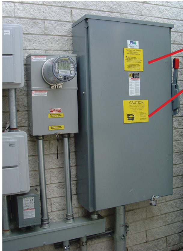
Power Shut-Off for PV System including Inverter
