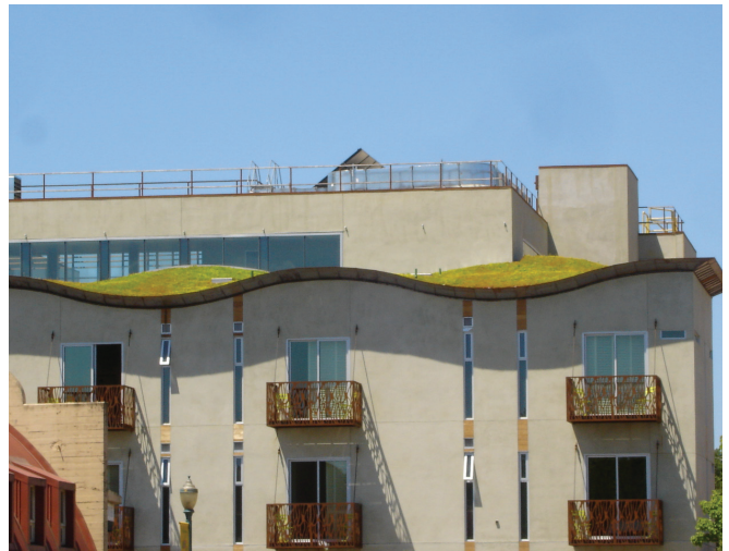
Growth media on a rolling-style roof
