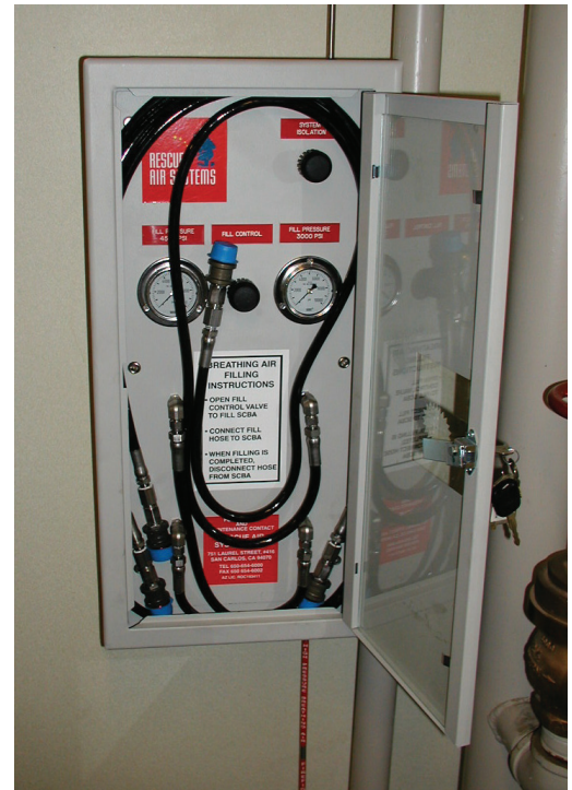
Firefighter breathing air replenishment system
