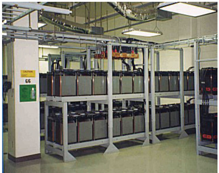
Battery room at a large data center
