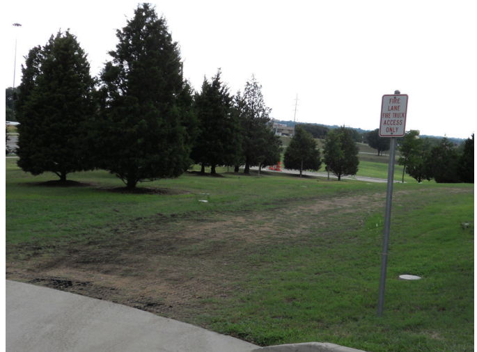
Permeable surface for fire department access road at a green campus. Note sign marking entrance and white markers outlining the roadway.
