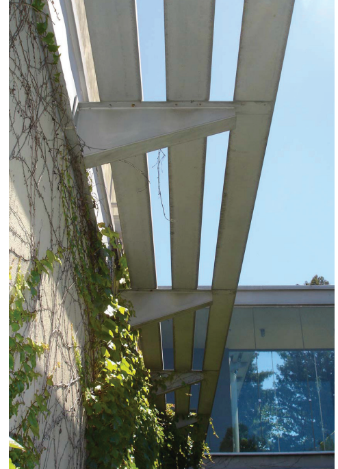
A green solar deflection system at the roof line provides shade to the building.
